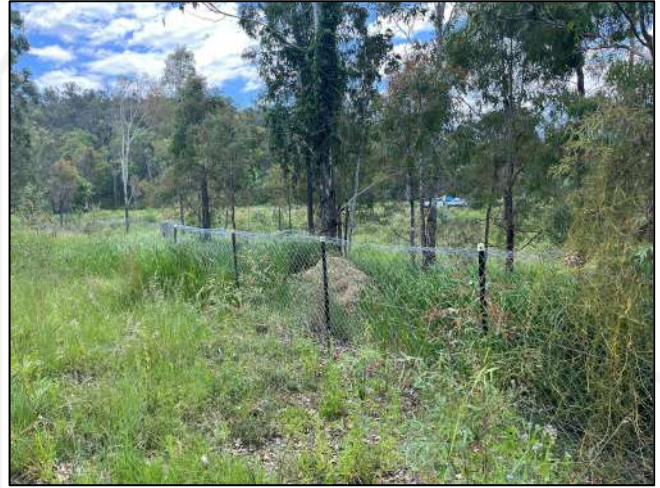
Photo Set 4: Temporary koala exclusion fencing along waterway corridor.
