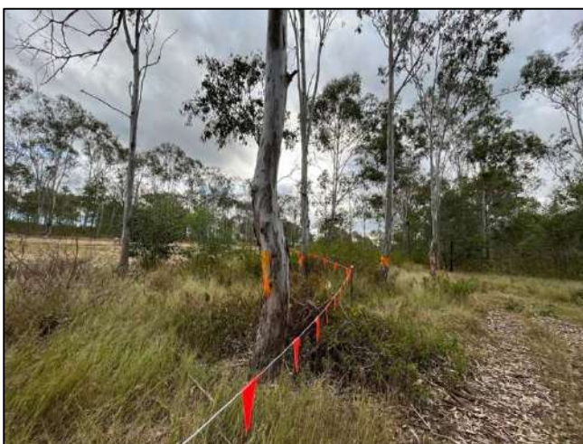
Photo Set 1: Temporary fauna friendly tree protection fencing.
