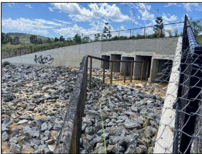
Photo Set 3: Fauna movement furniture within Barrams Road culvert crossing.
